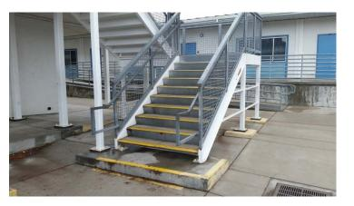
Photo -2 Stair and landing configuration at Building 16 does not appear to comply with current accessibility standards.
